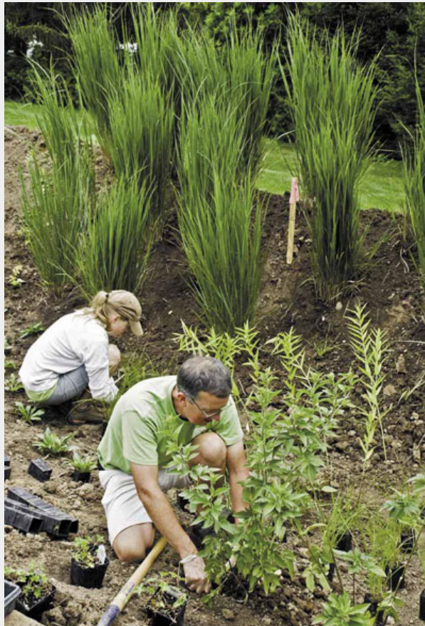
IMA horticulturists installed a rain garden on the property earlier this year. The rain garden is located adjacent to a parking lot and is designed to filter stormwater runoff to prevent pollutants from entering nearby waterways.
