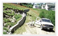
Notice the blue inclinometer between the soil engineers legs. There were originally several inclinometers installed on the slope and one on top of the slope by the house. All of them sheared off from the slope moving except the one by the house. It is being watched very closely, along with a new one that was recently installed on the other side of the house.
