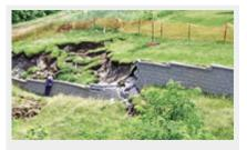
The dirt and sod has dropped substantially here, causing earthquake-looking "ravines" to open up and the wall to drop even further. The house at the top of the slope is in jeopardy. Inclinometers were installed at the beginning of the project to monitor slope movement. Photos courtesy of Turfmasters.
