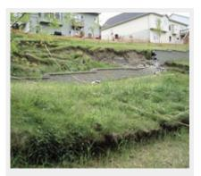
A substantial drop in this slope is evidenced by the wall that has dropped approximately 6 to 8 feet, as well as the dirt "ledges" caused by the earth shifting, moving and buckling as it slides further down the slope.
